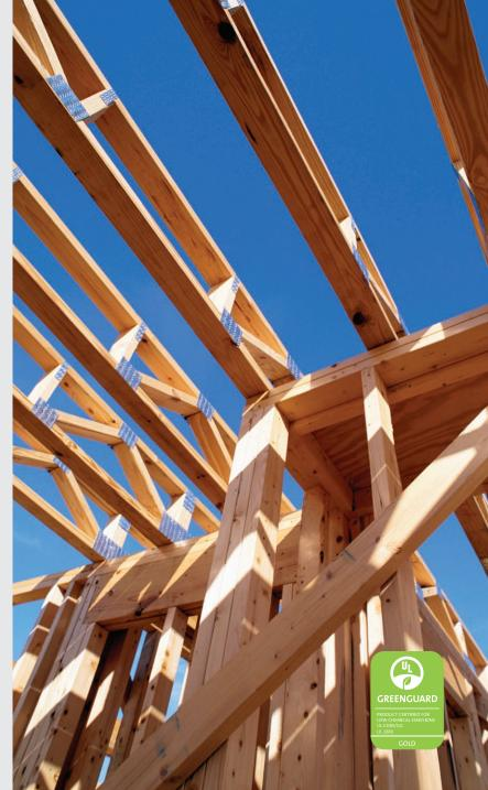
D-Blaze treated lumber and plywood is highly effective in slowing down the spread of flame and smoke development caused by fire. D-Blaze treated products show no evidence of significant progressive combustion after 30 minutes exposure to flame. In most applications, D-Blaze treated products offer a lower in-place cost than noncombustible-classified materials.
